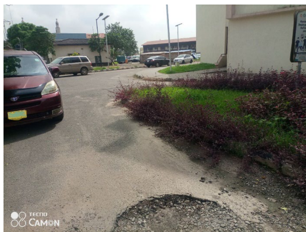
Figure 7: Unauthorized parking on the road (Source Authors' Field Work).
