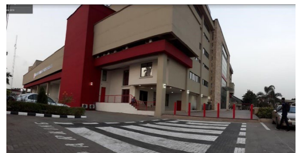
Plate 2. Image showing the façade of the Fountain of life church.
