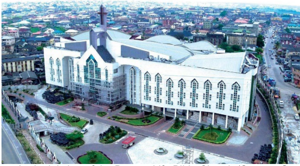
Figure 2. Aerial shot of the Deeper Life Bible Church (Source: Google)
