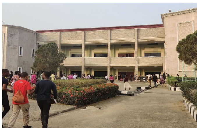
Plate 4. Image showing the permeable paved walkway around the Faith Tabernacle
