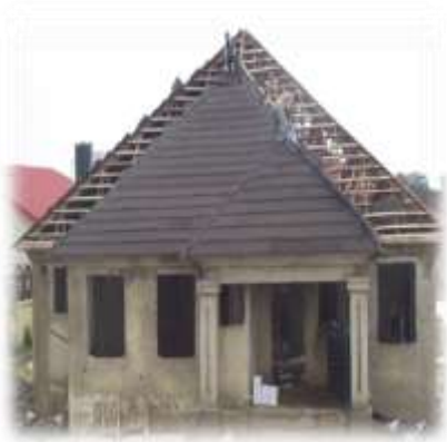
Plate 7: Roofing done same way as in the conventional method
