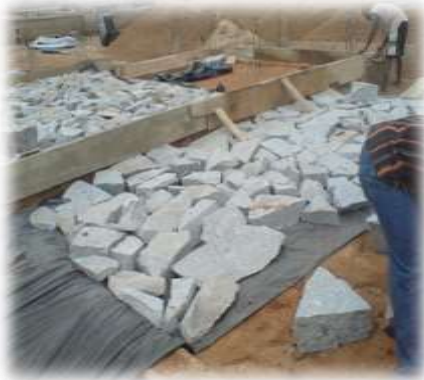
Plate 1: The foundation for EPS same as conventional method
