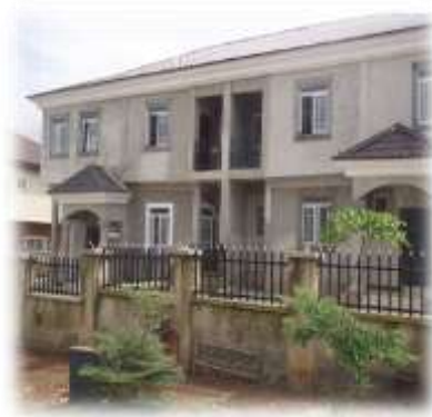
Plate 8: An EPS house ready for painting
