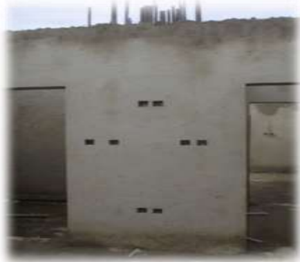
Plate 4: Same method of plastering for EPS and Conventional Sandcrete building
