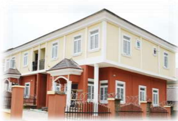
Plate 9: A Completed EPS House
