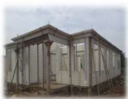
Plate 5: An EPS envelope ready to receive first stage of shortcreting (Spraying)
