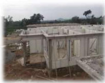
Plate 6: EPS Fascia (Cornices) are carefully strongly tied to the walls using wires and splice meshes
