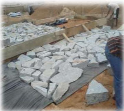
Plate 1: The foundation for EPS same as convectional method
