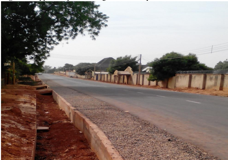
Figure 2: Type of Open Drainage in the Study Area
