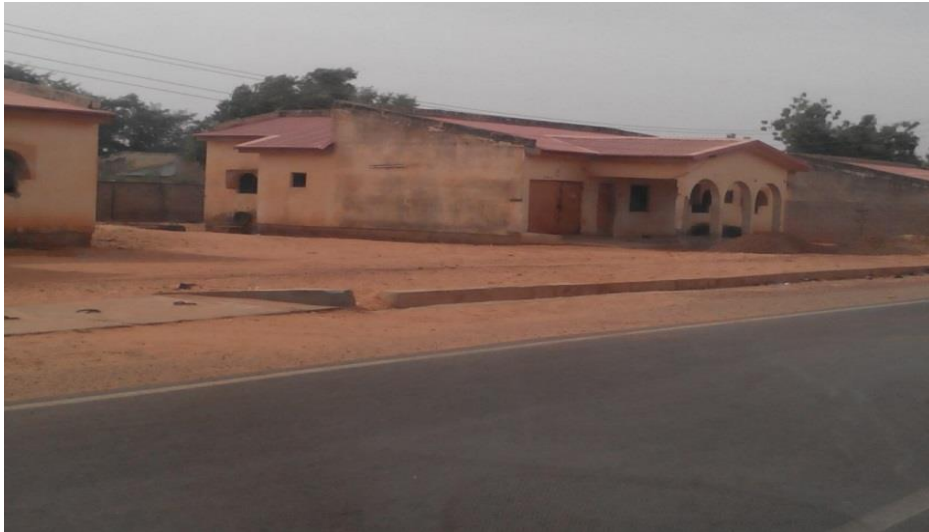
Figure 1: Blocks of Bungalows at the Gesse II Housing Estate Birnin Kebbi
