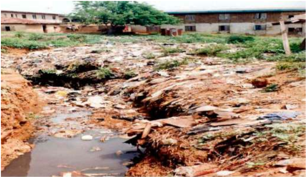
Plate 2: An unsightly drainage channel used as refuse dumps in the core of Ibadan, Nigeria. (Source: Laurent Fourchard)
