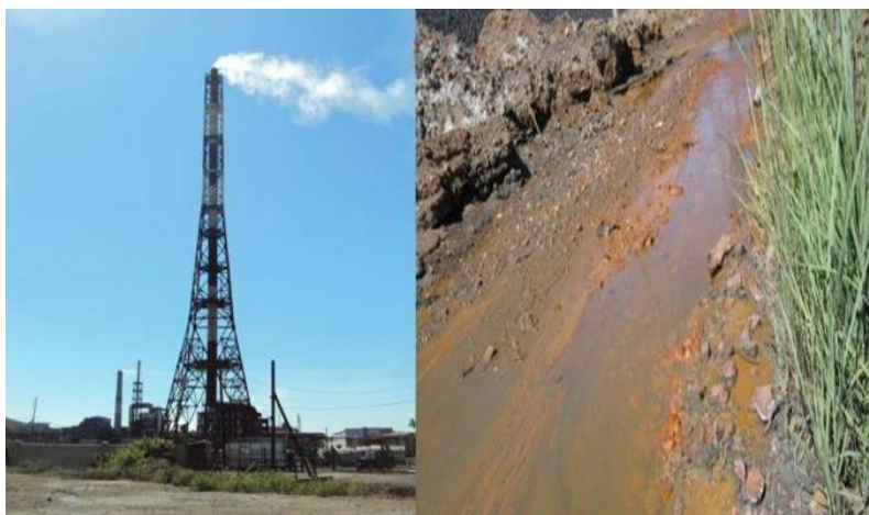
Fig. 1. Copper-Sulphuric plant in the city Mednogorsk.
