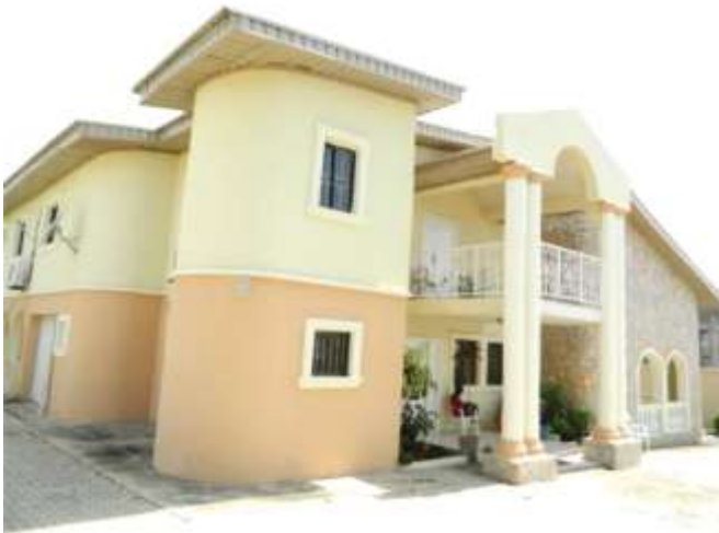
Plate: 1. A thin, protruding floor level definer (FLD) on a contemporary Ornamentation genre; in conjunction with the color differentiation application mark the floor level
