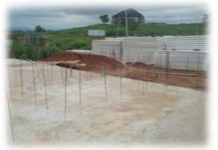
Plate 2: Starter Bars of Diameter 10mm are inserted At 500mm c/c before oversite concrete is cast
