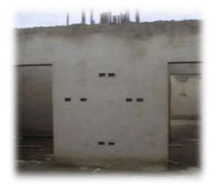
Plate 4: Same method of plastering for EPS and
